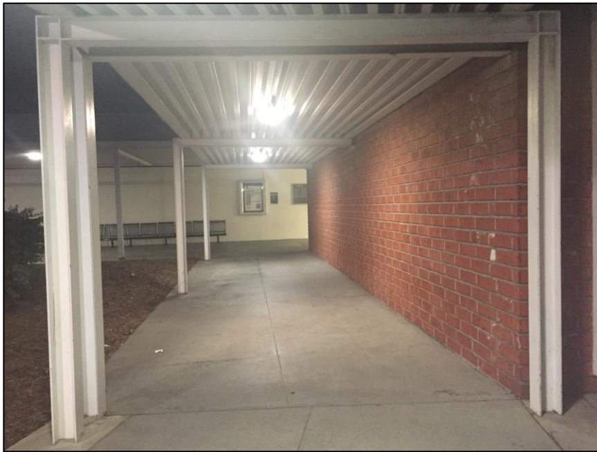
Figure 2. Moment frame. Photograph taken in the breezeway of Music building at California State University, Los Angeles
